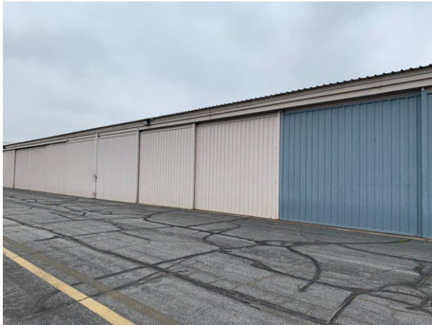
T- Hangar Row S
