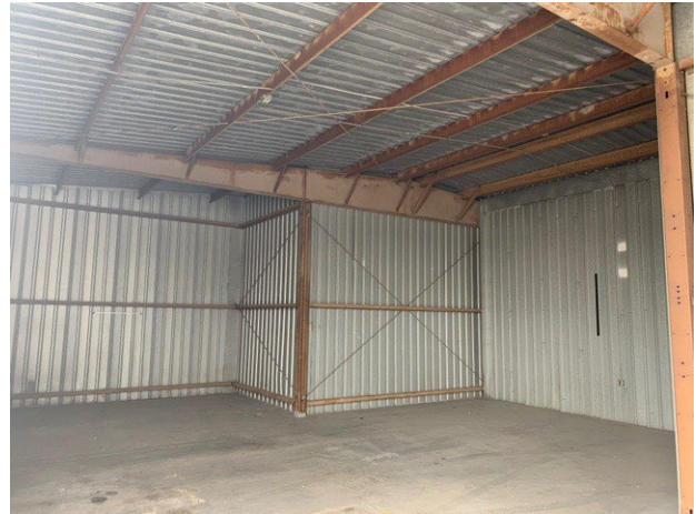
T- Hangar Row S
