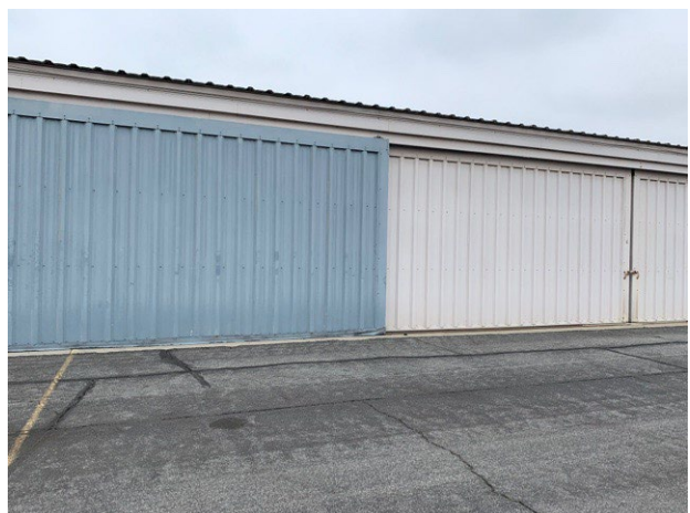
T- Hangar Row S
